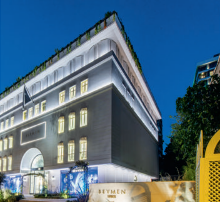
Beymen, Suadiye Architecture Office : HKMK Architecture Brand :Simes, Lasvit, Linea Light Group
