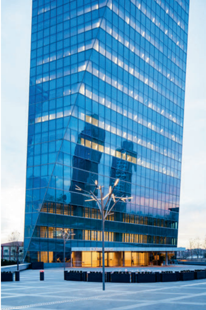
Finansbank, İstanbul Architecture Office : JBB Design Brand : iGuzzini
